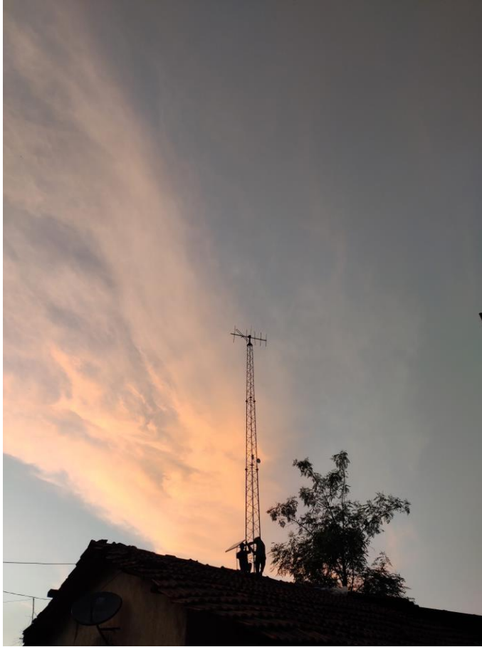
Figure 14: Deployment on the tower at Ramkhind.
